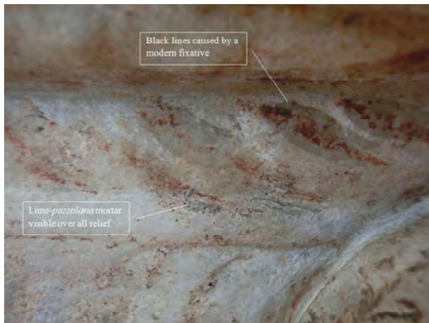
Fig. 7. Detail of the black lines attributed to modern restoration and of a modern mortar visible over the colour.
