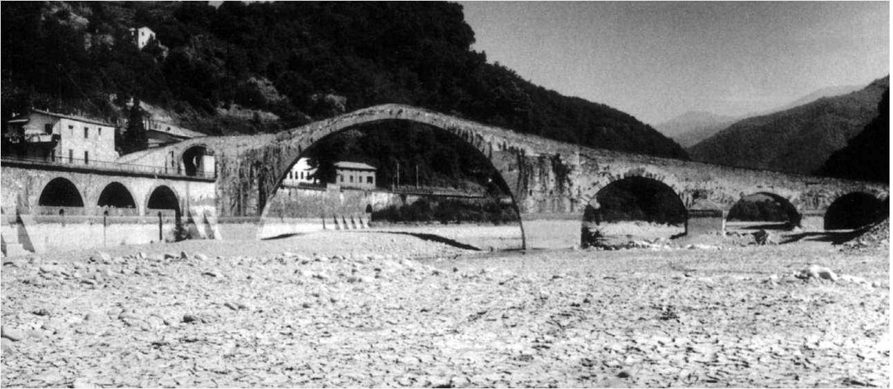
Figure 1. The Maddalena Bridge and adjacent railway.
