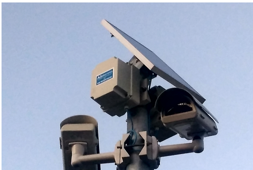
Figure 10. Picture showing the final field test installation.
