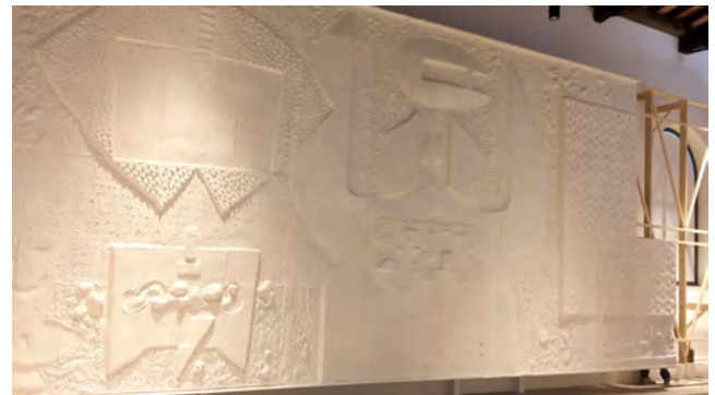
Figure 6: Assembly. The individual panels were mounted on a wooden frame before external coating and painting.
