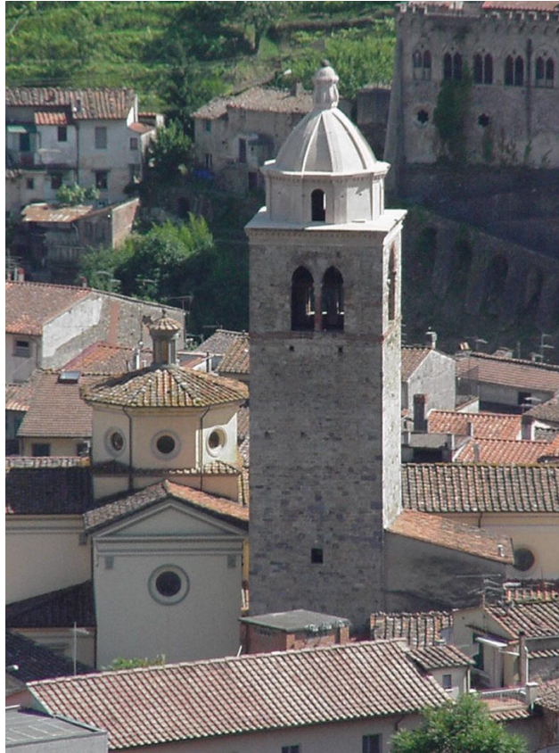
Figure 1. Buti's bell tower.
